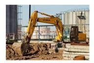
Excavation work presents a variety of hazards such as collapse of excavation, inrush or seepage of water and unplanned contact with hazardous services such as gas and electricity.
